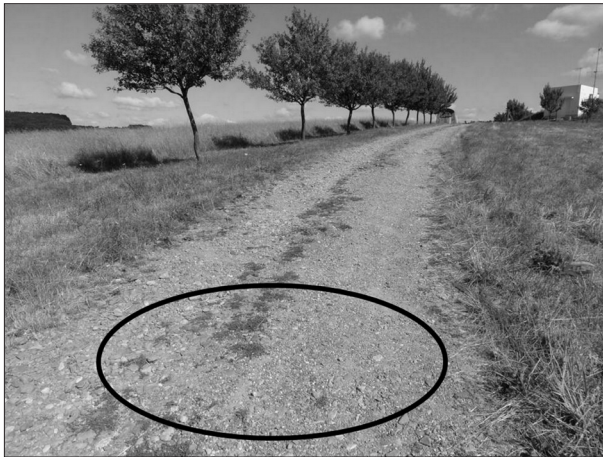
Fig. 12: The route to the cache – inappropriate, unpaved surface. Source: authors
