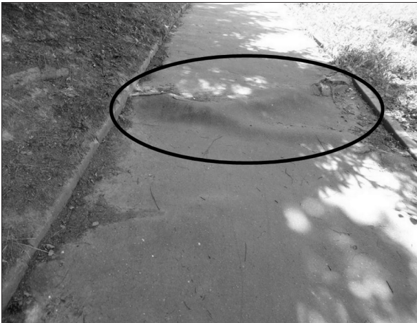
Fig. 8: The route to the cache – tar damaged by tree roots Source: authors
