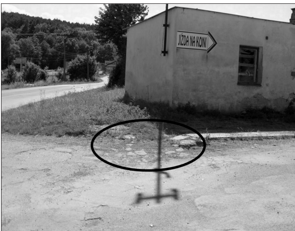
Fig. 10: Damaged surface does not allow wheelchair users to access the cache. Source: authors
