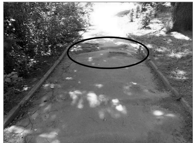
Fig. 15: Kerbs and damaged surface on the route Source: authors
