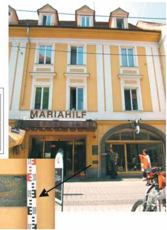
Fig. 29: Floodmarks on a house in the Austrian town of Schärding, commemorating historical floods on the Inn River (Photo: T. Strobl and G. Haimerl)
