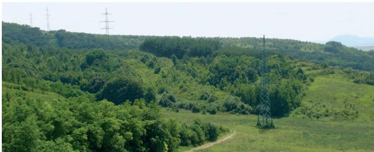
Fig. 12: High voltage power lines and forest aisle in Unit 3. (Photo: Markéta Flekalová)
