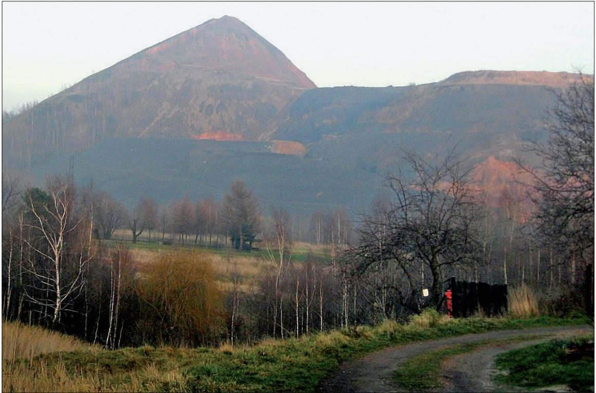
*Fig. 4: Coal mining waste dump Szarlota in Rydułtowy (USCB) – an example of conical dump (Photo Ł. Gawor)*
