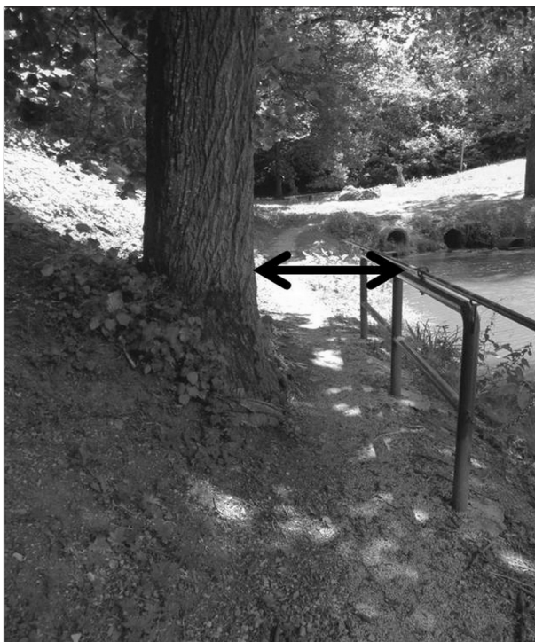
Fig. 16: The path narrowing to a width of 500 mm prevents a wheelchair user from passing. Source: authors
