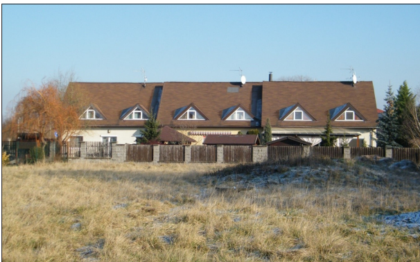
Fig. 8: Back-side of terraced houses from the early 2000s (C). They lie in the outer area, just next to the edge of the core area and next to a free plot. This is an extremely dense settlement, ANN below 11m Photo: Jiří-Jakub Zévl, 2019
