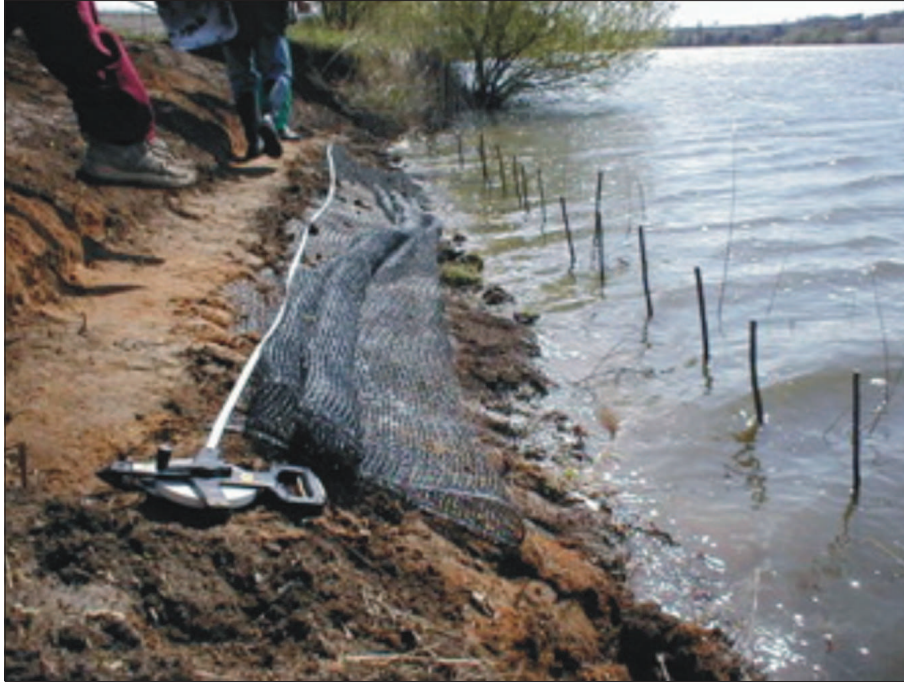
Fig. 6: Geonet was attached to the bottom range of Salix fluviatilis rods 0.7 m in length. Subsequently, geonet stabilized the slope of the same kind of willow cuttings in four rows. In conclusion, we stabilized the slope by a layer of soil of about 3 cm and sown grass mixtures (photo: M. Šlezinger)
