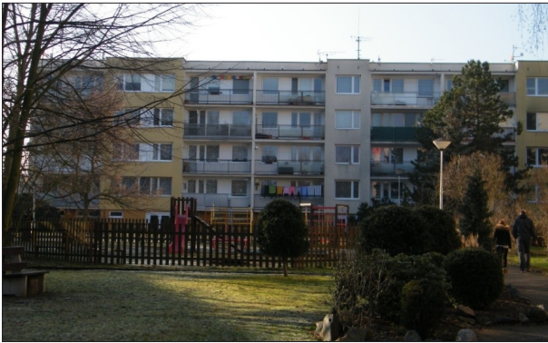
Fig. 6: Apartment house from the epoche of socialism (F), core area. The construction belongs to the average category of density (17.1 – 22.0m) Photo: Jiří-Jakub Zévl, 2019
