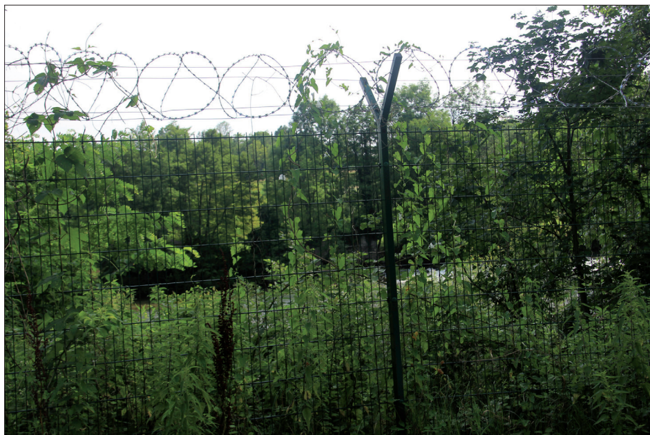
Fig. 5: The Slovenia–Croatia border barrier was erected near the Kolpa/Kupa River after the migrant crisis in 2015 Source: Matej Gabrovec, with permission
