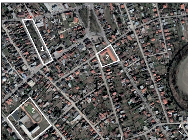
Fig. 4: Example of scattered layout of LC in Ivanka, Slovakia (main objects: 1 – recreational area, 2 – school) Source: Google Earth Pro, 22 June 2022
