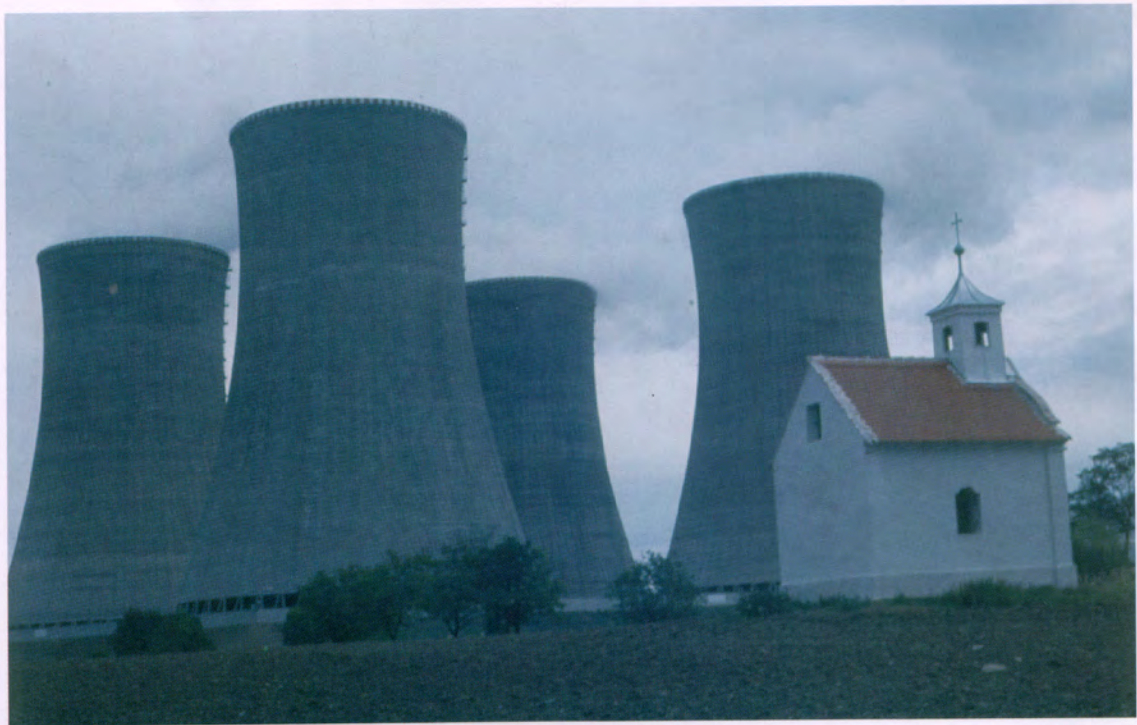
The past and the present: cooling towers of the nuclear power plant at Dukovany and the chapel of the destroyed village of Lipňany
