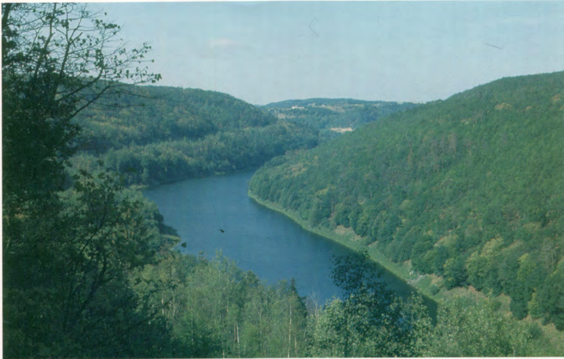
Mohelno: the lower water reservoir for the pump power plant Dalešice - a part of the power generation system Dukovany-Dalešice.
