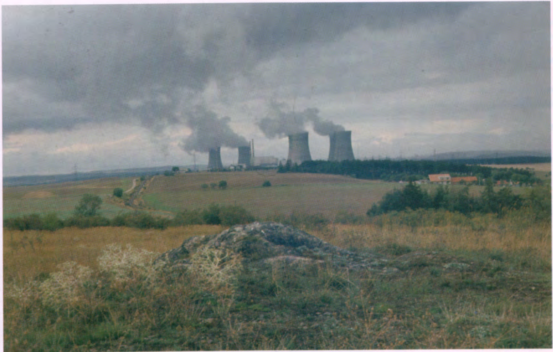
The nuclear power plant Dukovany - an anthropogenic element in the landscape a view from the East
