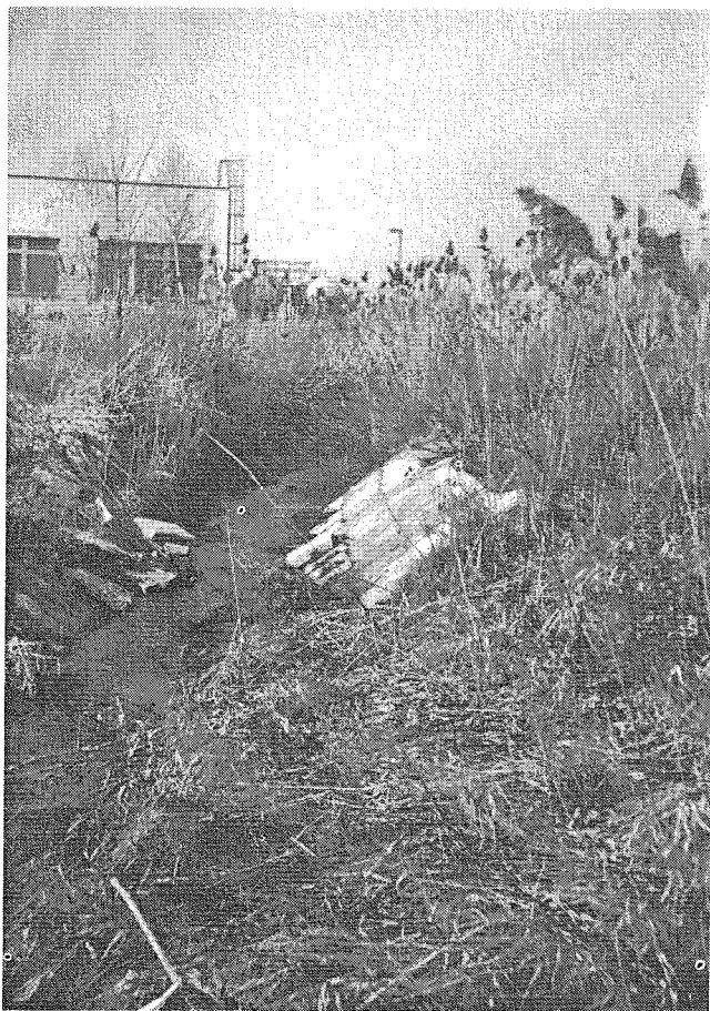
Fig. 3 Insufficient retention capacity of the landscape often results in increased erosion of water streams. The Daníř brook in the vicinity of an accumulation basin for irrigation near Chvalovice: at this place, high water damaged even the solid concrete pavement (Spring 1994).
