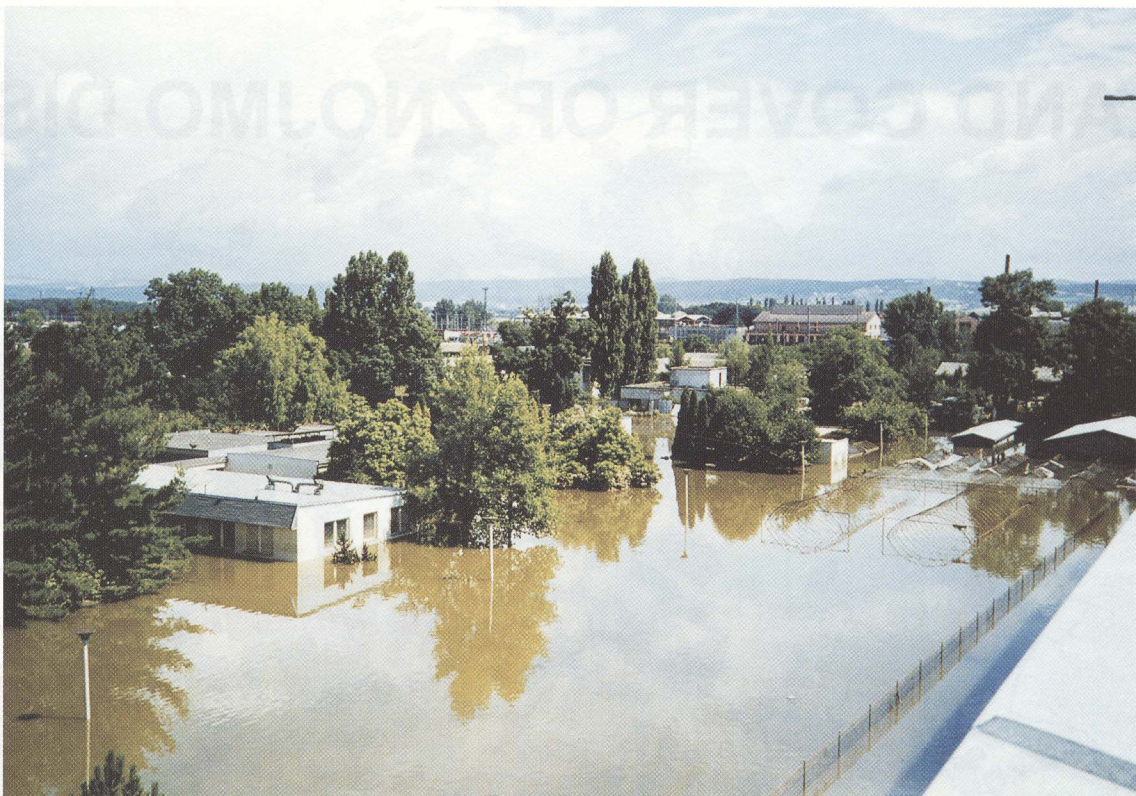
Aerial photograph of the Institute of Experimental Botany, AS CR in the town of Olomouc after the passage of flood wave
