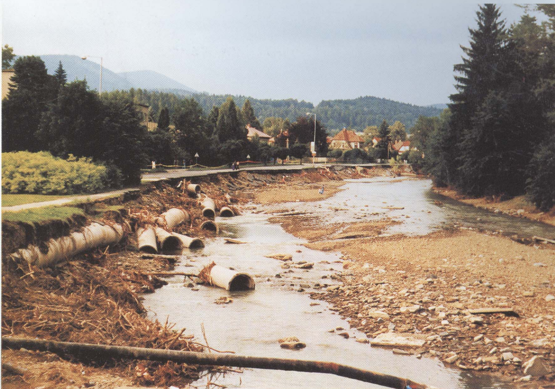
Rožnov pod Radhoštěm: destroyed bank and main road in the town centre after flood on the Rožnovská Bečva River. (Thursday, 17 July 1997)
