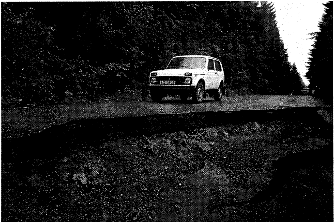
Fig. 5 Damaged road in the escarpment part of the large band slide on the Dušná Hill (732 m) near Vsetín town. Photo: O. Krejčí
