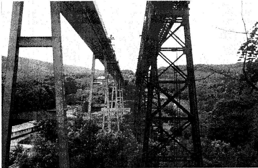
Fig. 8 The railway bridge across the Jihlava River valley is called the Ivančice Viaduct. At present there are two bridges. The old bridge was constructed in 1870 and the new one after more than a hundred years, in 1978. The necessity of construction of a new bridge demonstrates some difficulties with stability of supporting systems of the older one and close proximity of both structures with disturbed stability shows questionableness of this site for foundation of structures in general. Photo M. Hrádek.
