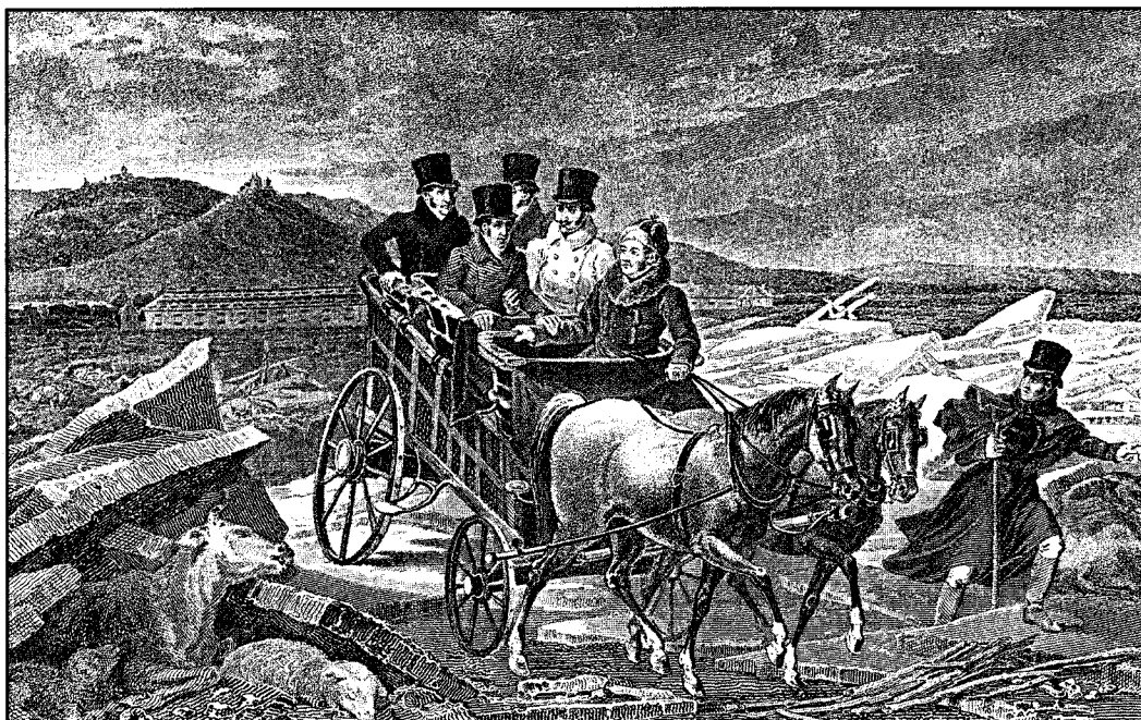
Figure 5: Royal Prince Archduke Ferdinand with his companion inspects the landscape on the Moravian Field short after the flood in 1830.
