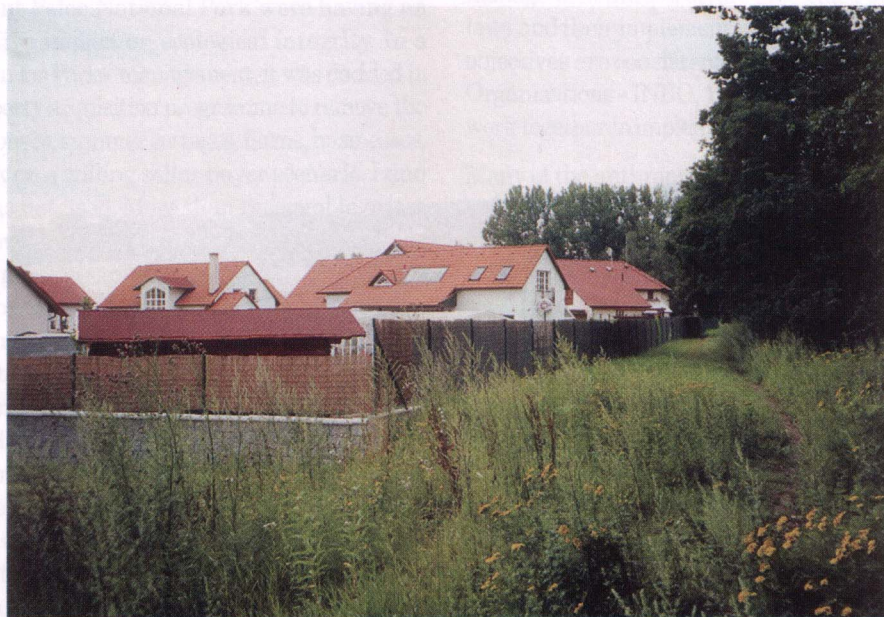
Fig. 2: New housing development in 100 year flood zone initiated prior to the 1997 floods showing illegal positioning at Litovelské Pomoraví Landscape Protected Area
