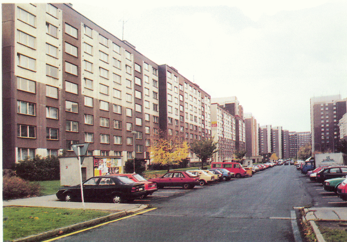
Complex home building (Frýdek-Místek, housing estate Slezská)
