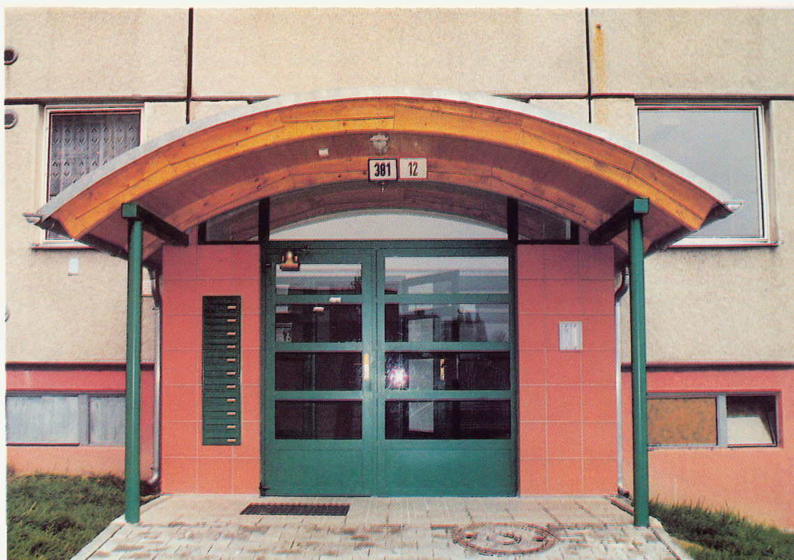
Front door of a panel apartment house after successful reconstruction (Havířov, housing estate Šumbark)
