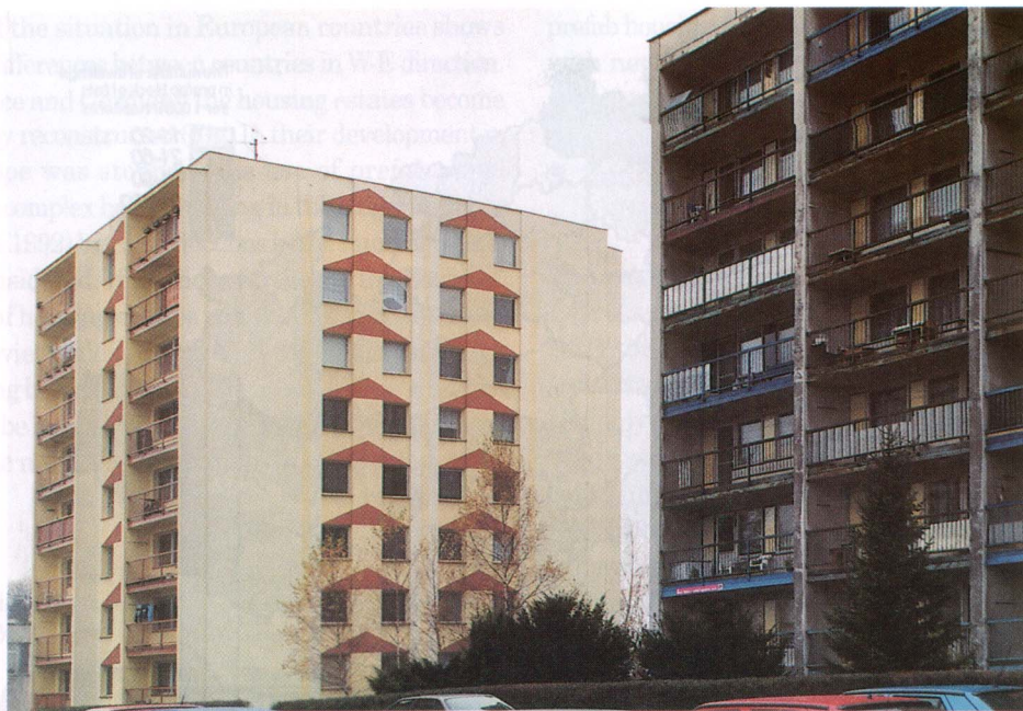
Fig. 5 Example of successful humanization of housing environment of one of the prefab houses (Haviřov, prefab housing estate Šumbark, 2001). Photo: E. Kallabová
