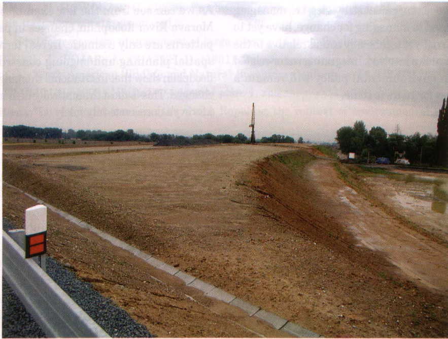
Fig. 4: Questionable new highway by-pass constructed perpendicular to the floodplain
