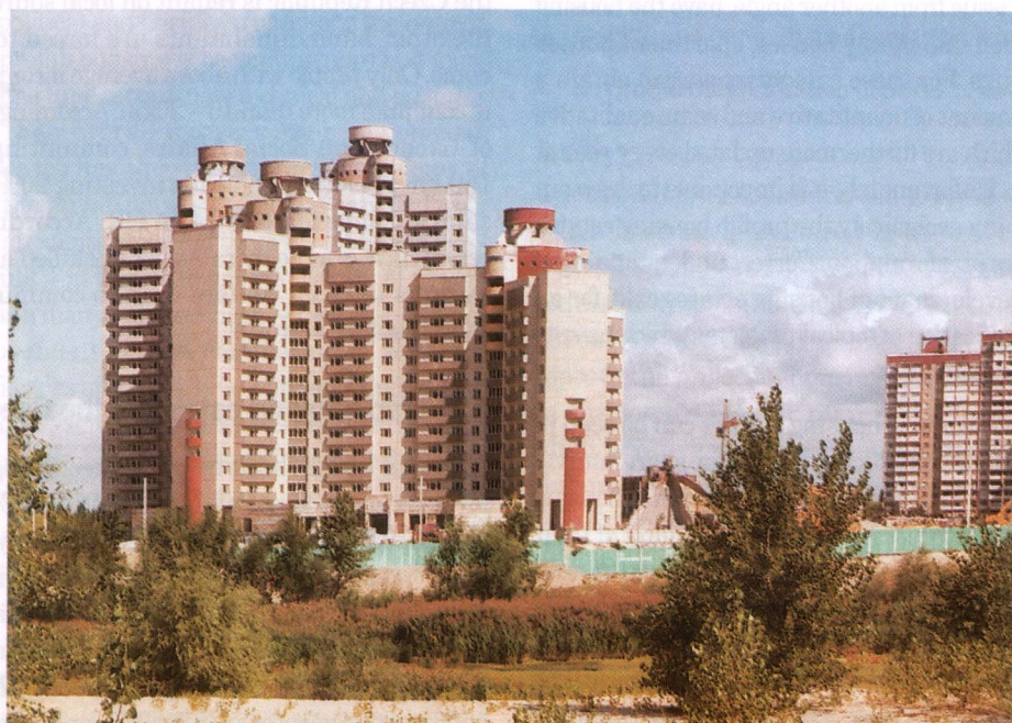
Fig. 2: Building of new prefab housing estate (Ukraine, Kiev, housing estate Livoberezhna, 2000). Photo: E. Kallabová
