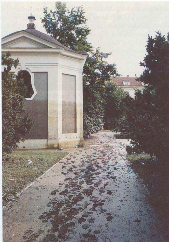
Fig. 12: The chapel of Saint Teresa in Vojan's municipal park (Prague Lesser Town) 17 August 2002, three days after culmination with maximum height of flood water still apparent on her walls. (Photo H. Váňová)
