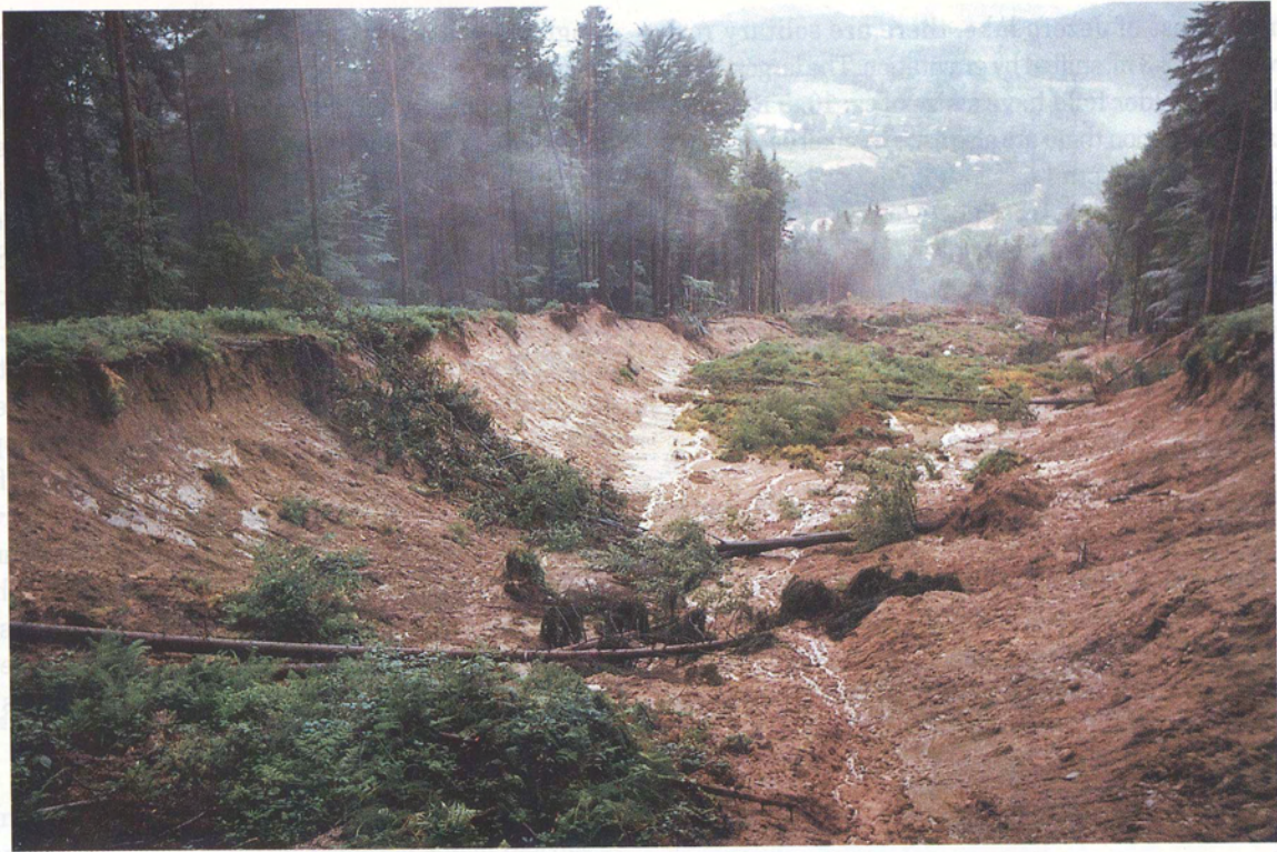
Photo 2: The Bystřička landslide - the upper part of locality is modelled by earth flow (state to July of 1997). Photo O. Krejčí.
