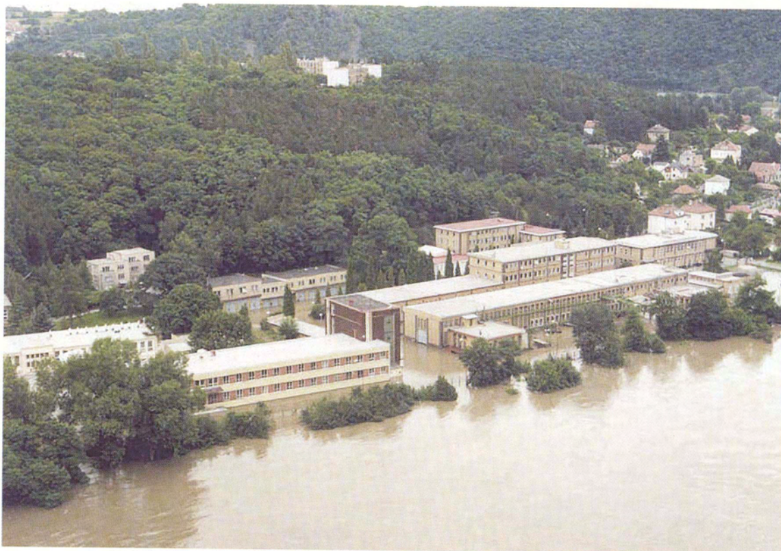
Flooded premises of the Institute of Nuclear Research Řež, a.s., Nuclear Physics Institute AS CR, and Institute of Inorganic Chemistry AS CR in Řež north of Prague on the right bank of the Moldau River on 14 August 2002.
