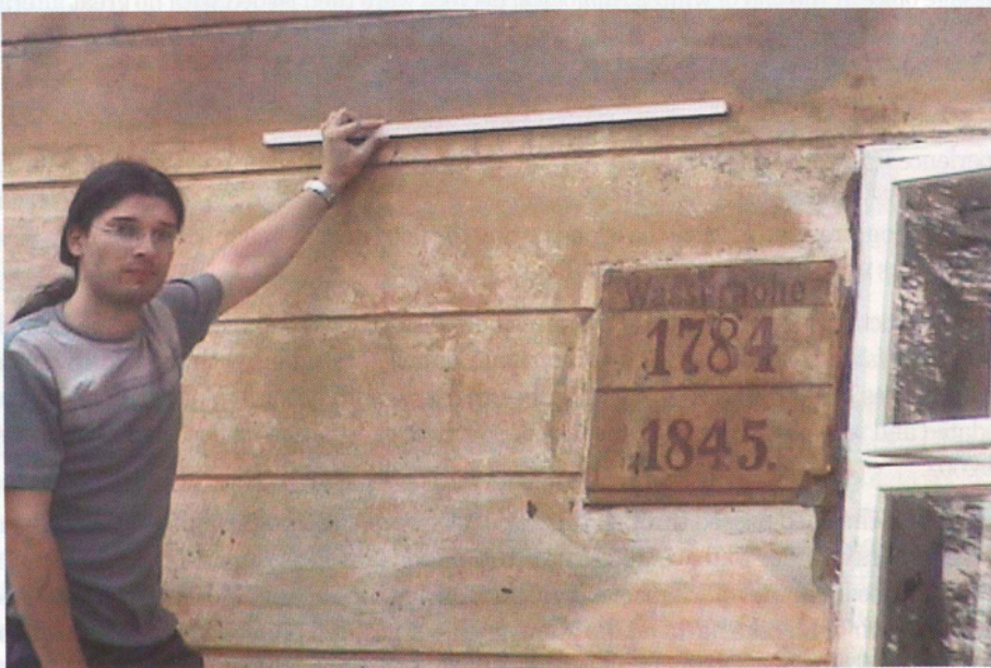
Fig. 10: A house on the left embankment of the Moldau River on the Kampa near the Charles Bridge in Prague with culmination marks of two big historical floods. The flood in August 2002 surmounted the culmination from March 1845 by 75 cm and that from February 1784 by 55 cm. (Photo J. Kubát)
