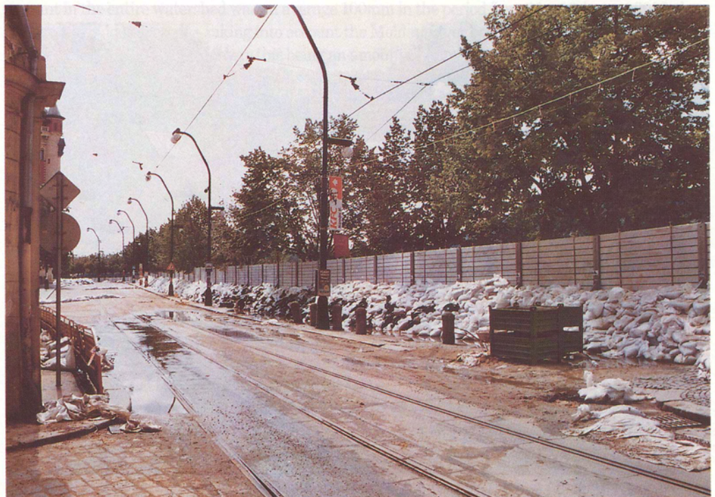
Fig. 5: Mobile dike walls in the lowest part of Smetanovo nábřeží (embankment) on the right bank of the Moldau R. near the Charles Bridge in Prague. (Photo H. Váňová)
