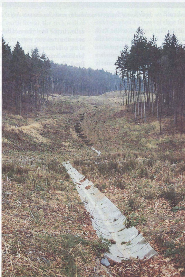
Photo 3: Reclamation in upper and middle part of the Bystrčička landslide (state to April of 2000). Photo O. Krejčí.
