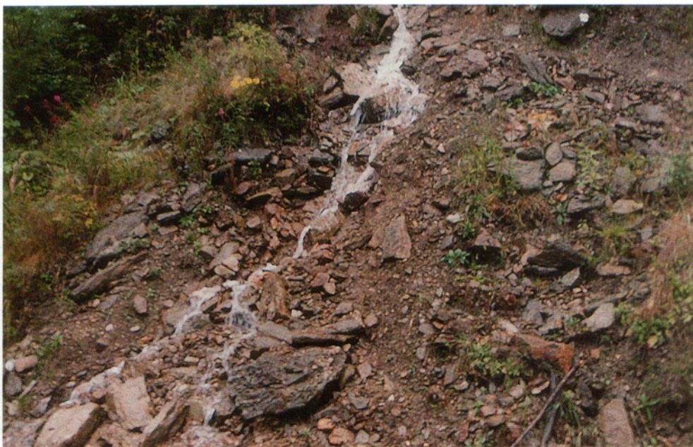
Photo 4: The unprotected sides of newly constructed forest road at the foot of eastern slope of Hučivá Desná valley built of mica schist scree cause natural hazards of rapid water erosion and gravity-controlled mass movement. Photo M. Hrádek
