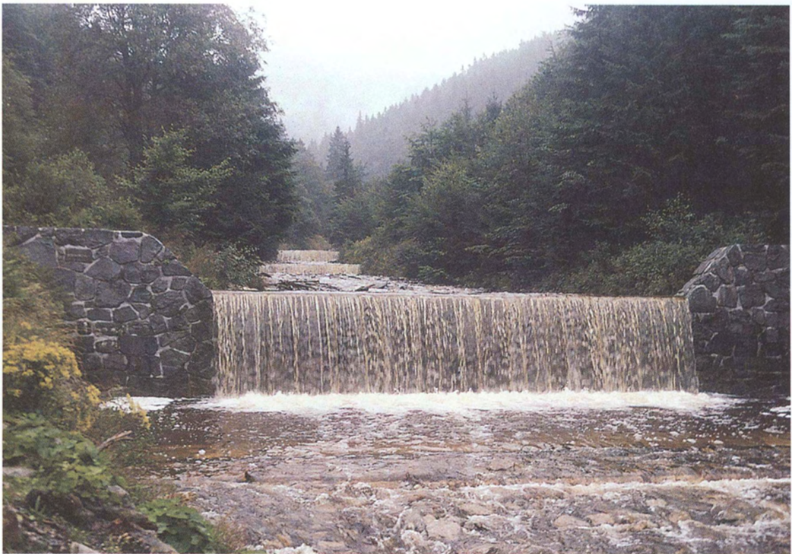
Photo 5: Channel of the Hučivá Desná R. is in its middle reach regulated by weirs and dams.
