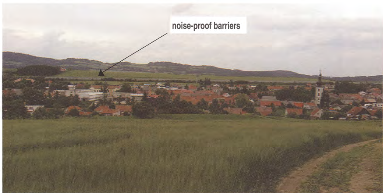
Fig. 4: Village of Měřín in 2004 (highway D1 with noise-proof barriers). Photo P. Trnka
