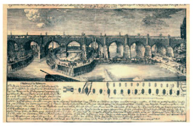
Fig. 8: Repair of the Charles' Bridge in Prague after the flood of 1784. Copper engraving by K. Salzer, original size 28.5 x 45.5 cm (Museum of the Capital of Prague).
