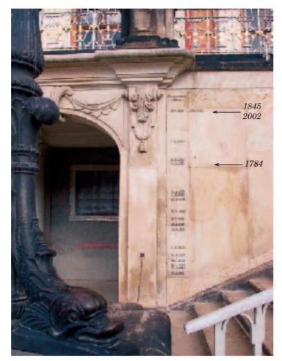
Fig. 11: High water mark of the extreme from 1 March 1784 on the water pavilion of Pillnitz Chateau near Dresden on the right Labe (Elbe) R. bank, and a comparison with the floods of 2002, 1845, 1890 and 1862 (Photo: U. Grünewald).
