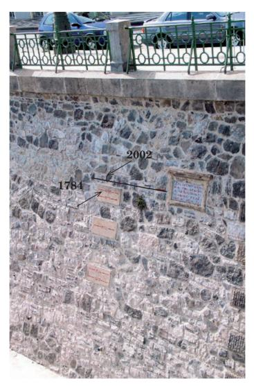
Fig. 6: Comparison of the Vltava (Moldau) R. culmination in August 2002 (Fig. 5) with floods in 1784, 1845, 1862, 1876 and 1872 (Photo: D. Karfík). With respect to the fact that the quay wall was under construction in 1870 - 1877, the extreme of September 1890 – the last high water before the case of 2002 - is not included.
