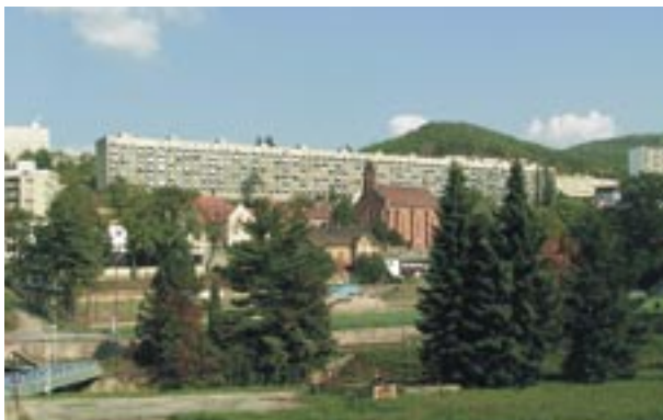
Fig. 5: Adamov (Czech Republic - population 5,000) is an extreme case of industrialized town. Prefabricated houses built in the 1970s stand in a sharp contrast to the rest of the original village represented by the Church of St. Barbara. The whole scene is surrounded with valuable forests. (Photo: E. Kallabová)
