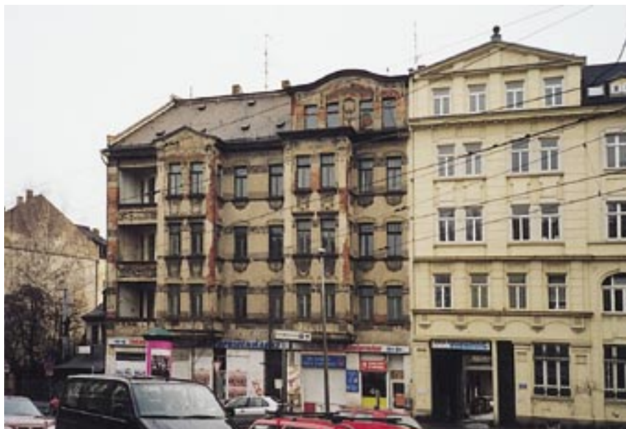
Fig. 3: Area under re-urbanization in Leipzig: dilapidation houses contrast with reconstructed housing stock. (Photo: A. Vaishar)
