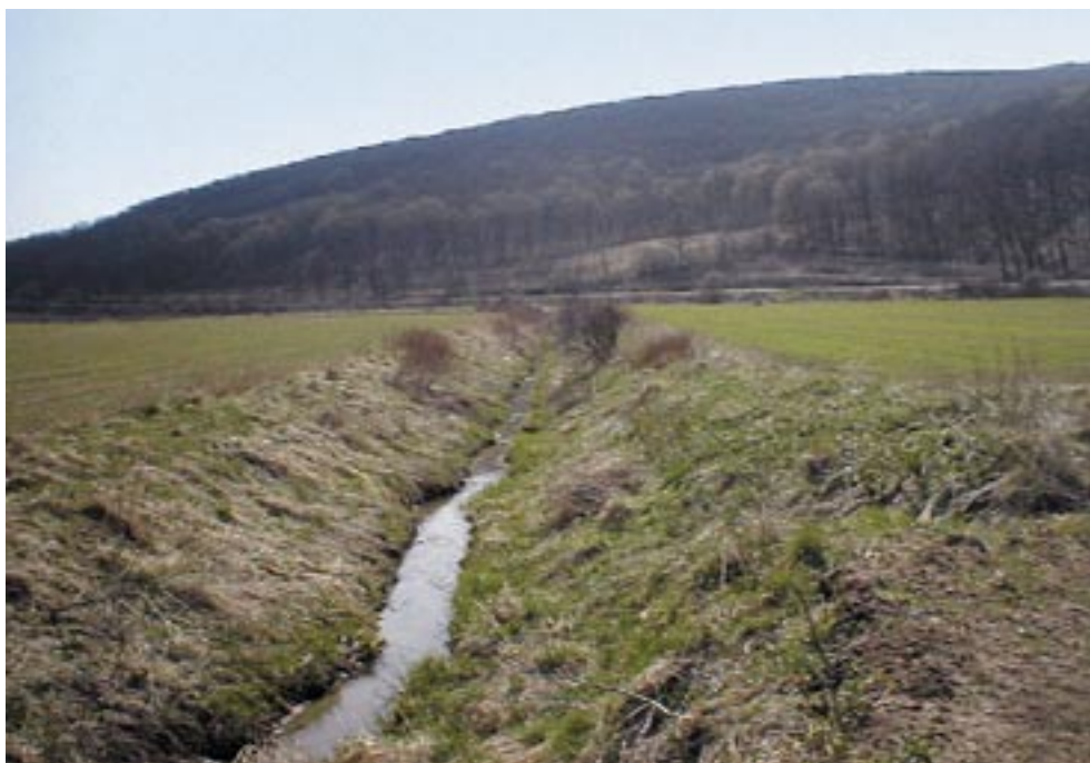
Fig. 2: Modified channel of the middle part of Haraska stream (Photo: H. Svatoňová, April 2003)
