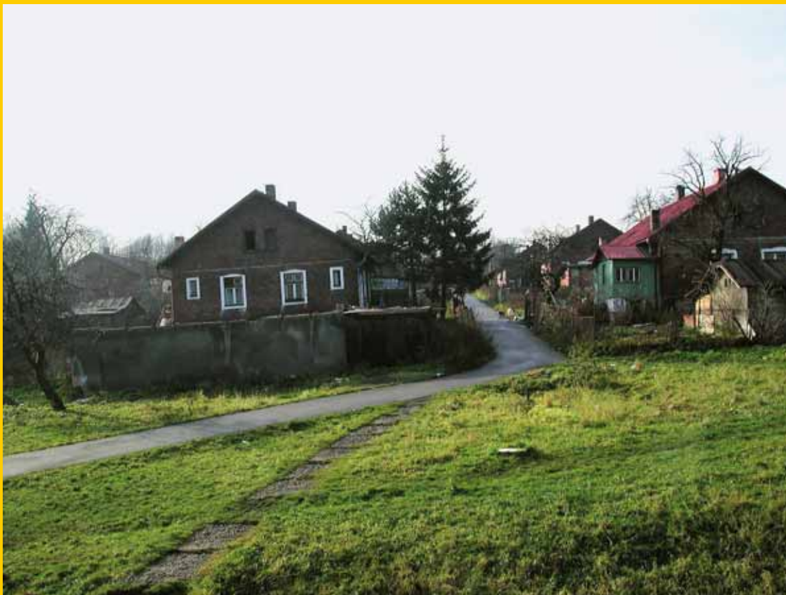
Fig. 5: Workers' colony in the outskirts of Olová – situation until 2004 (Photo O. Mikulík)
