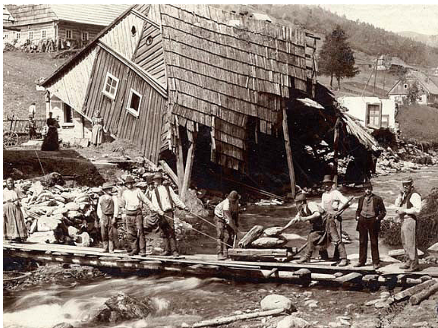
Fig. 11: Damages after the flood on the Úpa River in July 1897 in the village of Velká Úpa (Archives of P. Scheufler)
