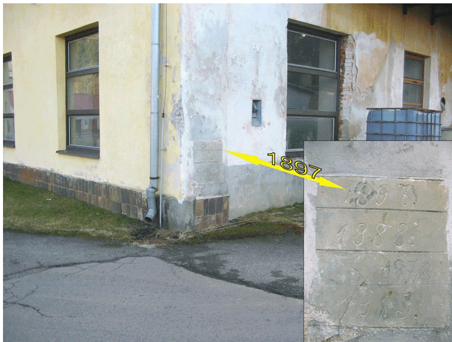
Fig. 4: Flood marks on the Jizera River in Jablonec nad Jizerou (Photo: J. Luštinec)
