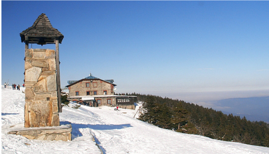
Fig. 2: Jiří's Lodge at Šerák on the main tourist ridge trail – the oldest stone lodge in Hrubý Jeseník built after the original lodge had burnt down 1894 (Photo J. Havrlant, 2008)
