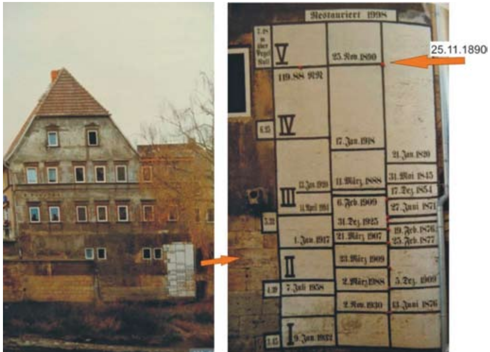
Fig. 8: A residential building in the town of Camburg on the bank of the Saale River. Flood-marks on its wall were restored in 1998. They clearly indicate that the highest recorded flood waters were here on 25 th November 1890, which reached 7.18 meters above the water-gauge zero point during the culmination (Photo M. Deutsch)
