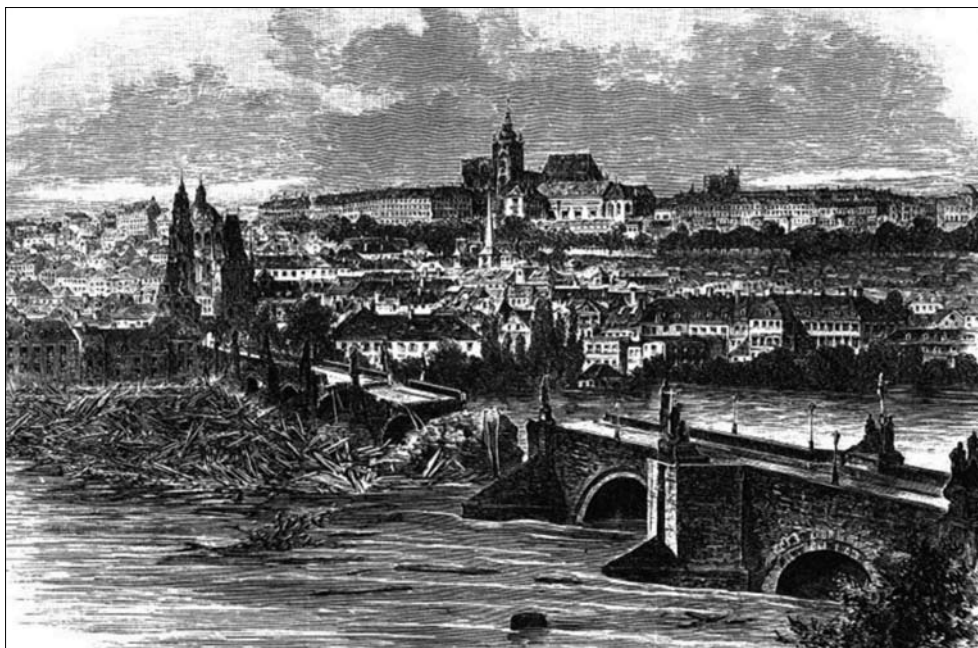
Fig. 2: The catastrophic flood on the Vltava/Moldau R. in September 1890 was the last one to damage the Charles Bridge in Prague. Two of its arches were torn apart on the third day of flooding – 4 September 1890 – as a result of the accumulation of a large amount of logs (Collection of M. Deutsch)
