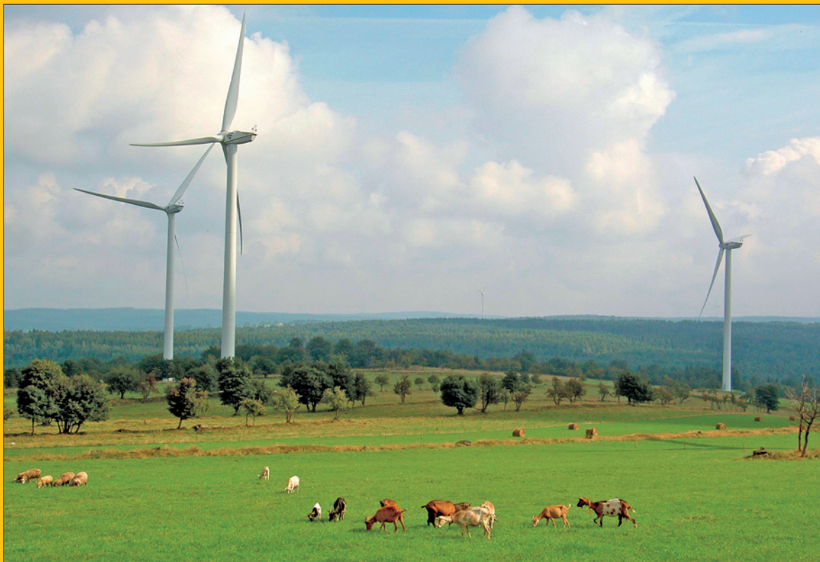
Fig. 5: Wind farm in Nová Ves v Horách (district of Most) – an alternative energy path for coal mining region (Photo: B. Frantál)
