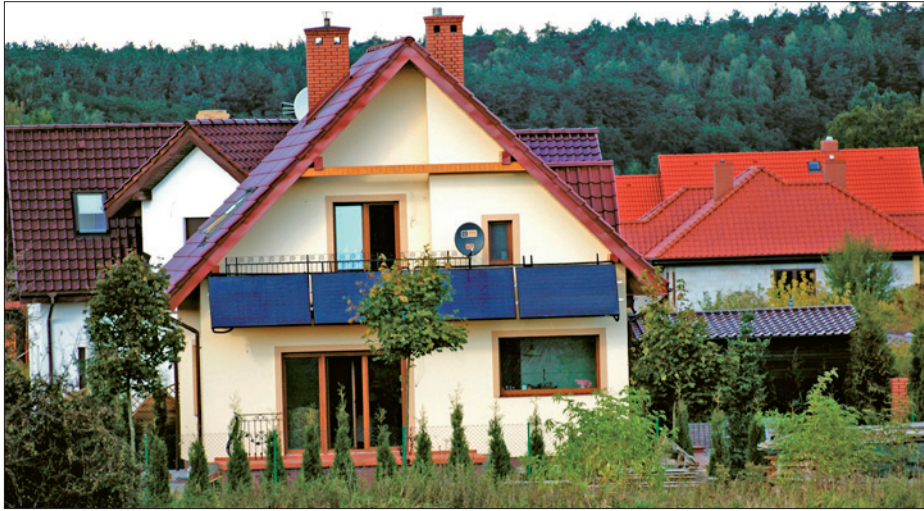
Fig. 3: A single family-house with solar collectors in Czarnowo – a suburban area of the Bydgoszcz–Toruń agglomeration (Kujawsko-Pomorskie Voivodship) – an example of the BAPV system. Source: author
