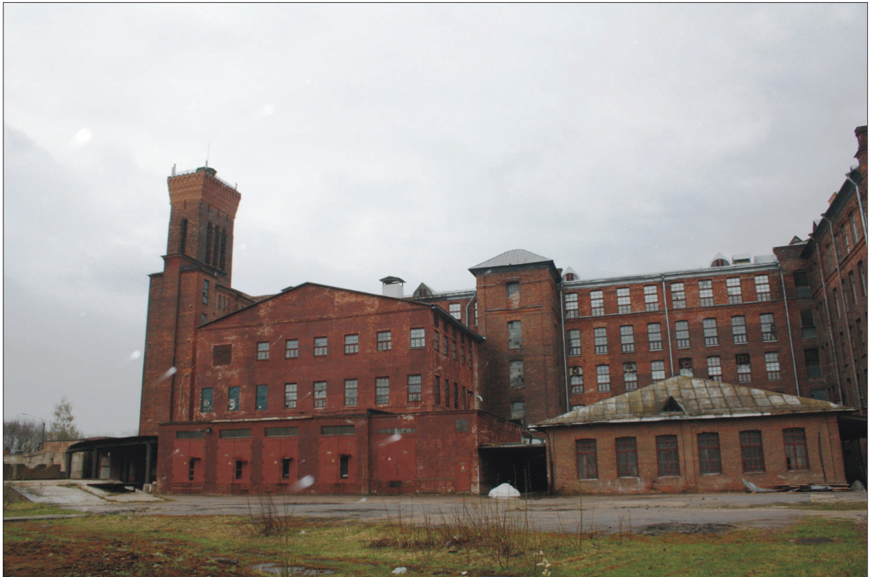
Fig. 7: Derelict buildings of the textile factory in Kreenholm island Narva (Estonia) (Photo: J. Tintëra)
