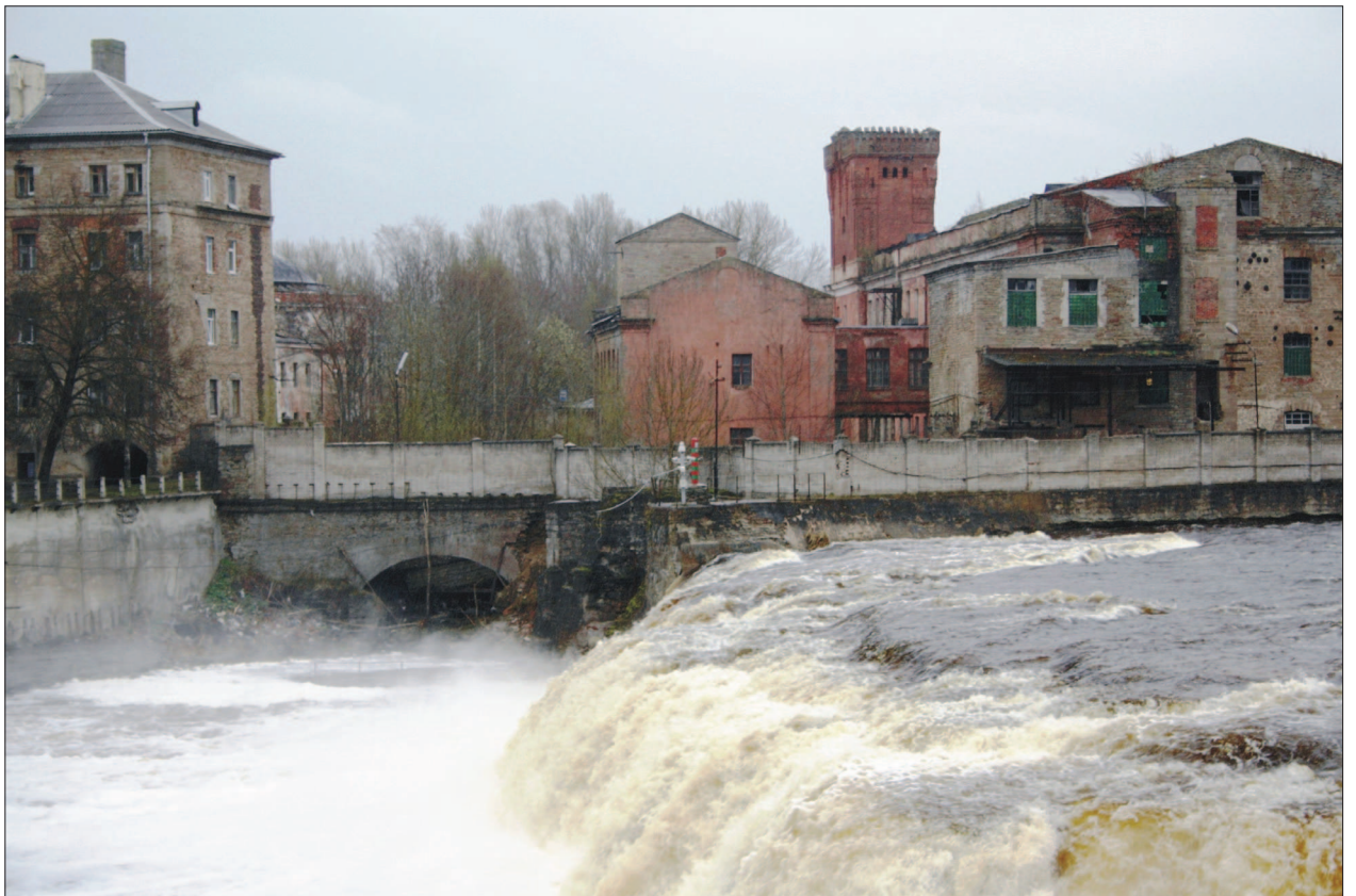
Fig. 8: Former textile factory in Kreenholm island (Narva, Estonia) - view from the East (Photo: J. Tintëra)
