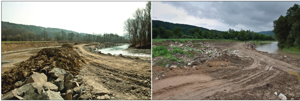
Fig. 8: An example of non-environmentally friendly river management. Channel lateral movement and bank erosion in the meander loop was stopped by the dike and the channel was shifted to the position before the flood event (left image). The inter-dike area close to the eroded bank was filled downstream by construction waste (right image). Despite these measures, channel migration continues. Photo: M. Rusnák
