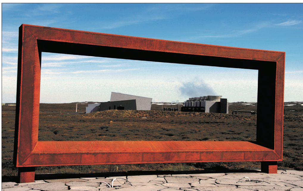
Fig. 4: The geothermal picturesque? New power station at Teistareykir, NE-Iceland Photo: Karl Benediktsson
