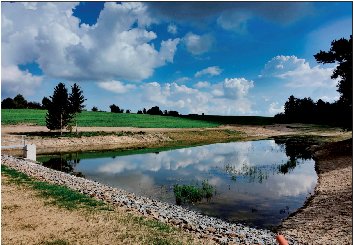
Fig. 11: Newly restored man-made pond for water retention in the landscape. It was built on the location of the drained historical pond in Šebestěnice (Czech Republic) (Photo: J. Frajer, 2021)
