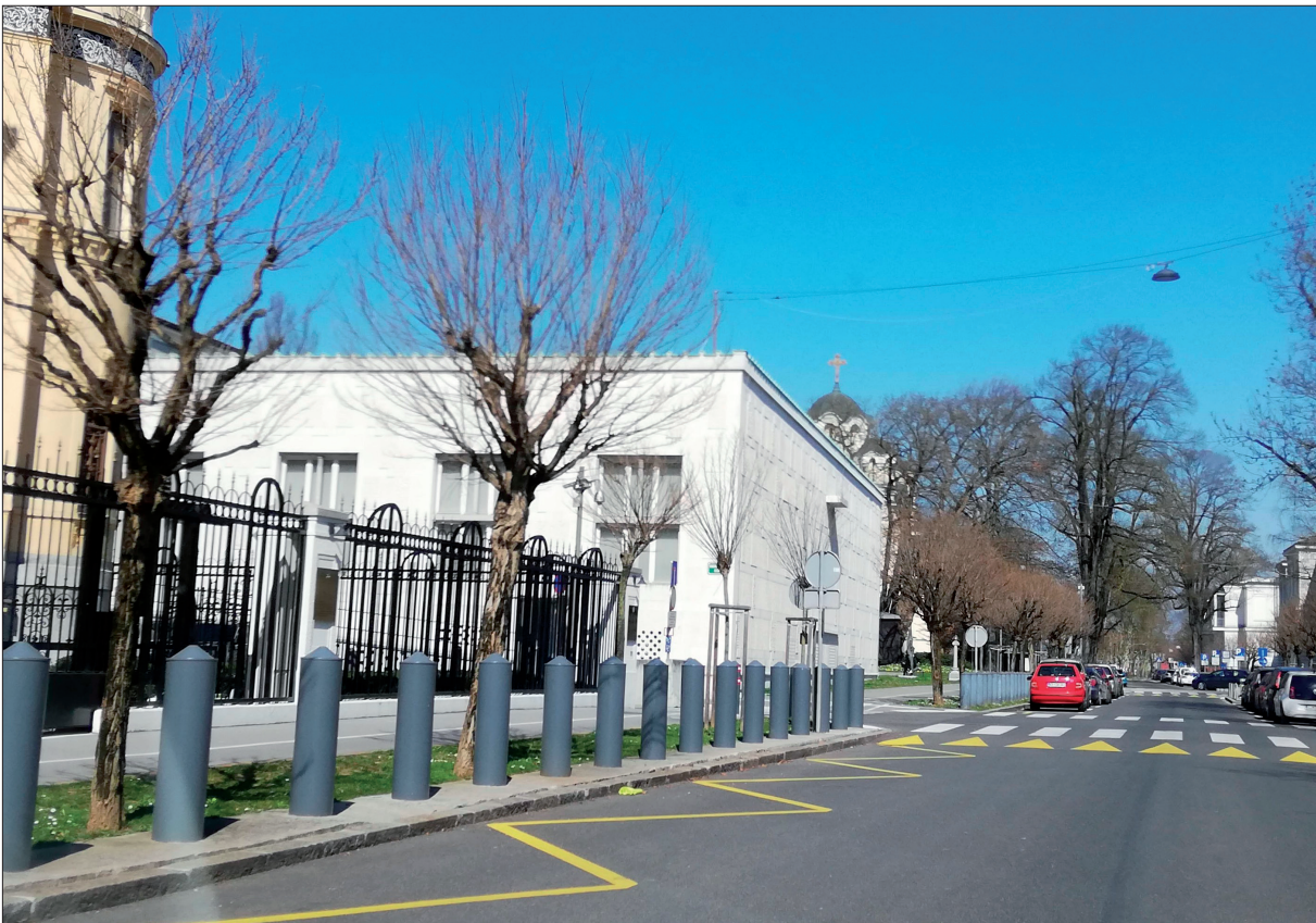
Fig. 11: Reinforced barrier of the USA Embassy parcel on Prešernova Street in Ljubljana (Photo: B. Komac)
