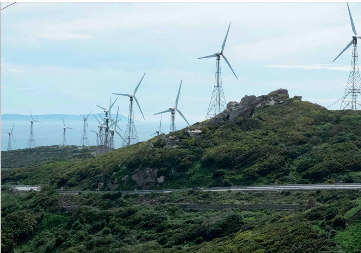
Fig. 9: Wind farm El Cabrito, implemented in 1993 (Tarifa, Spain), before repowering (Photo: M. Frolova)
